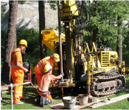
Figure 3. Side view of the borehole location
