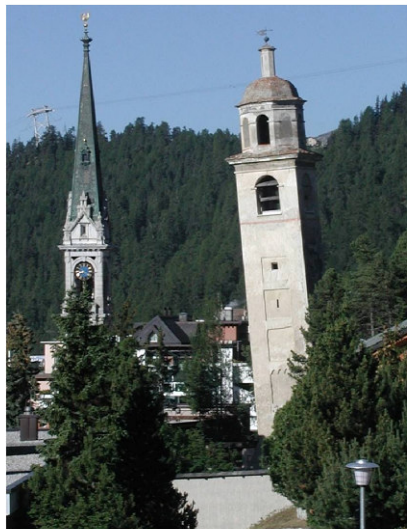
Figure 4. The leaning tower of St. Moritz
