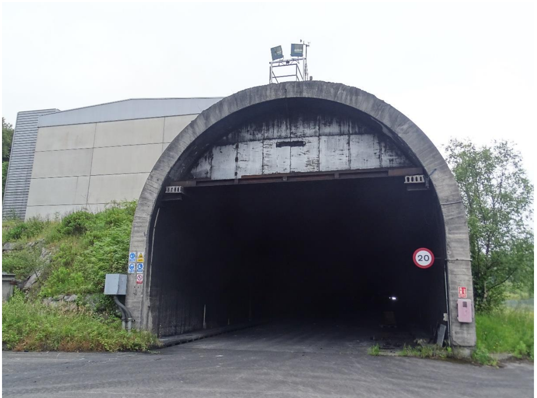
Figure 41: North portal San Pedro des Anes with false ceiling
