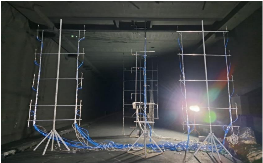
Figure 47: Air velocity and temperature grid installation
