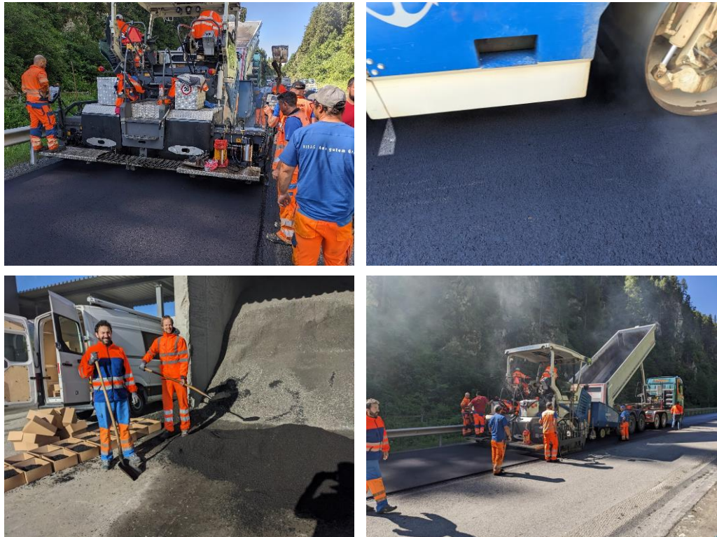
Figure 106: Construction of the AC 8 S pavement in the Charnadüra test section
