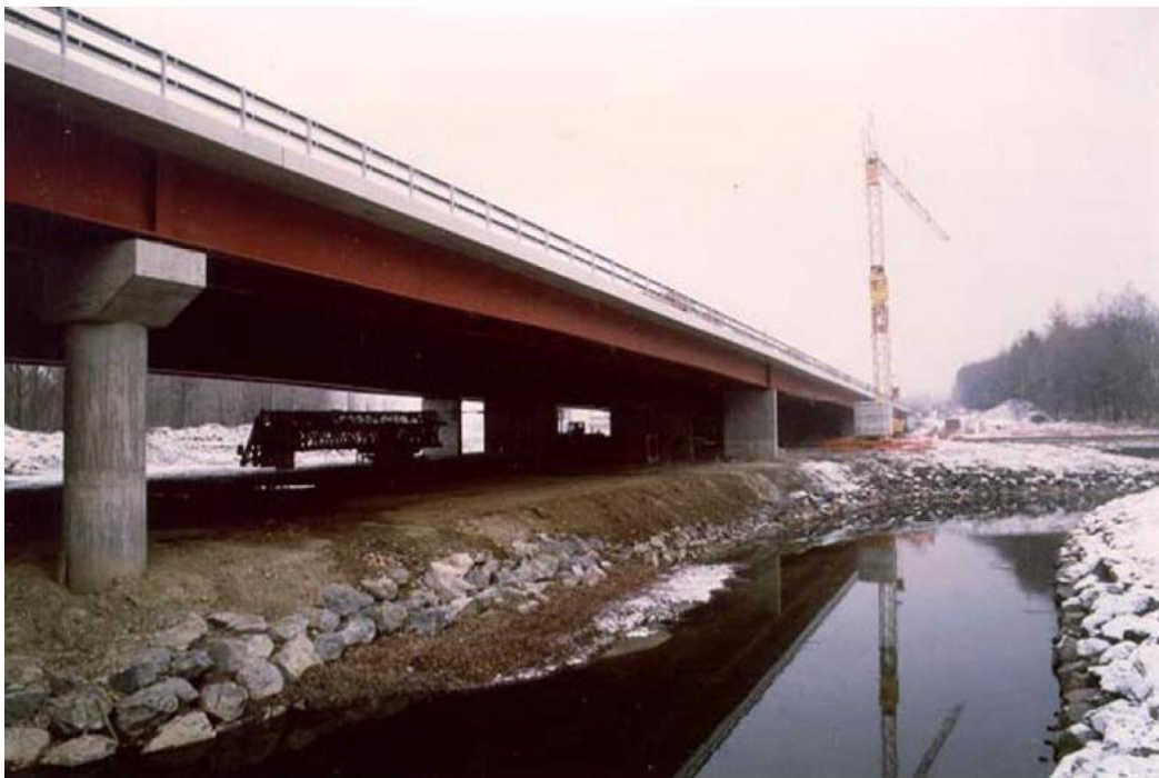
Fig. 50 The Venoge bridge, Ecublens (Switzerland).
