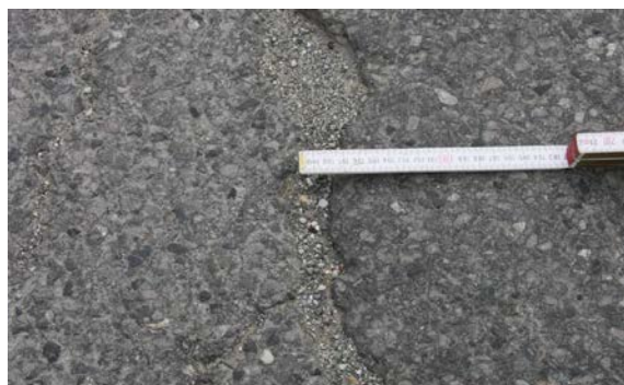
Brückenende Detail links
