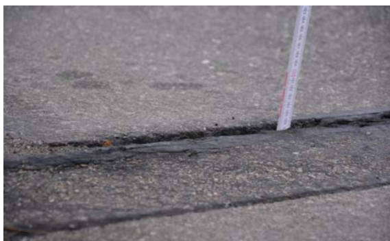
Brückenende Detail links
