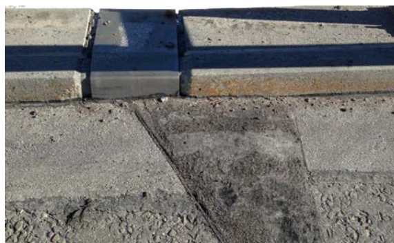
Brückenende Detail links
