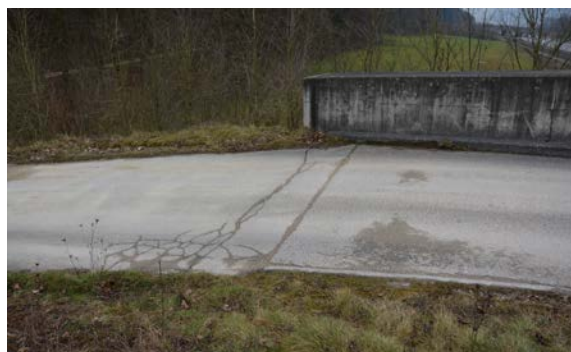
Brückenende Detail links
