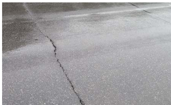
Brückenende Detail links
