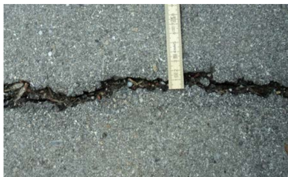
Brückenende Detail links
