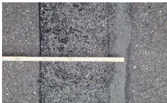
Brückenende Detail links
