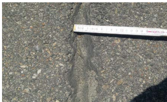
Brückenende Detail links
