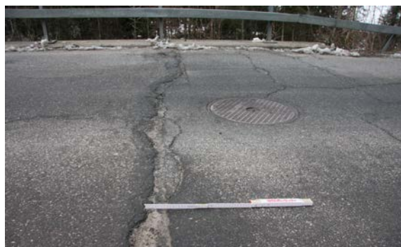
Brückenende Detail links
