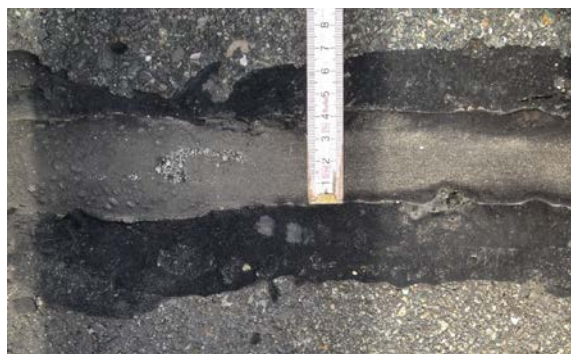
Brückenende Detail links
