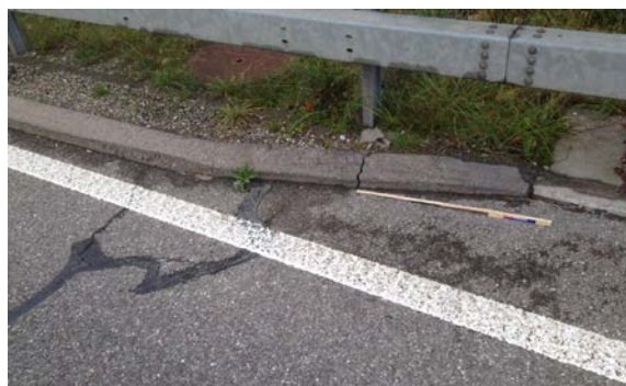
Brückenende Detail links
