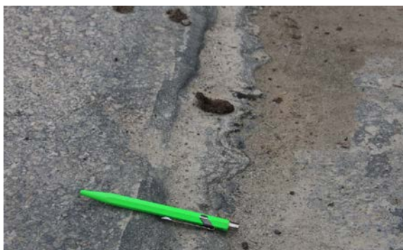
Brückenende Detail links
