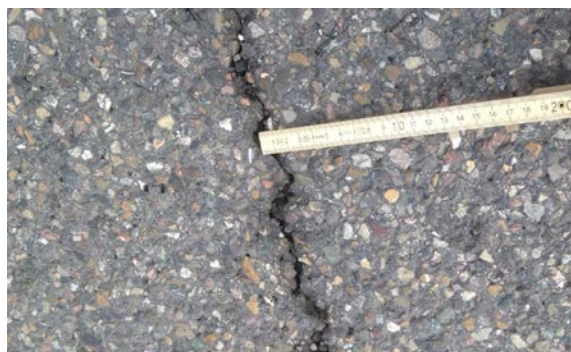
Brückenende Detail links
