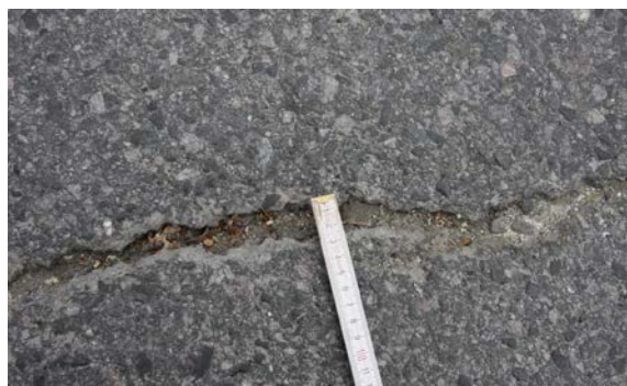
Brückenende Detail links
