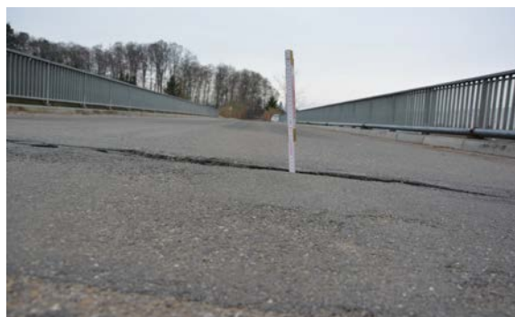
Brückenende Detail links
