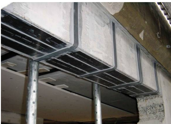
Figure 1.3 Beams reinforced with bonded CFRP strips (CCLab) [11]
