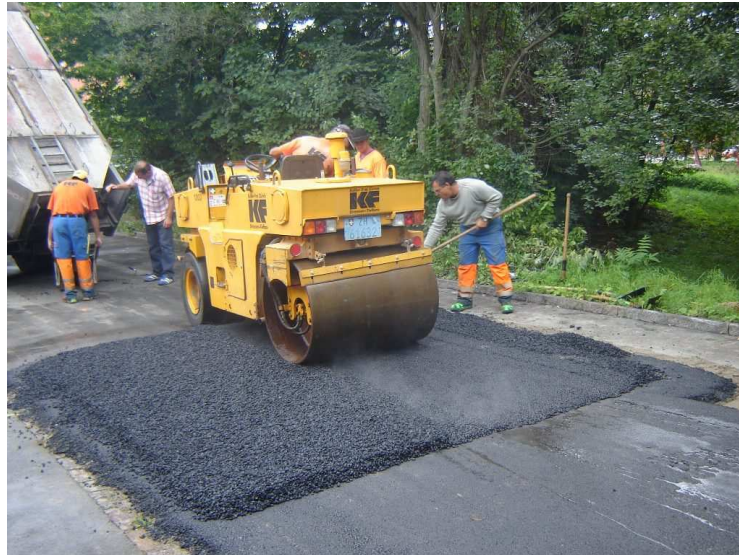
Fig. 3.10: Preparation of the two pavements investigated with MMLS (AC bottom right, PA centre, work in progress).
