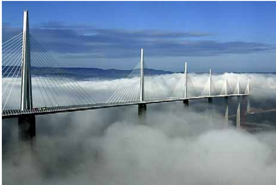
Figure 10: Cable-stayed bridge (Millau viaduct, France).
