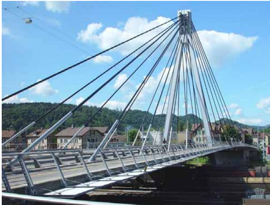
Figure 60: Stork Bridge in Winterthur.
