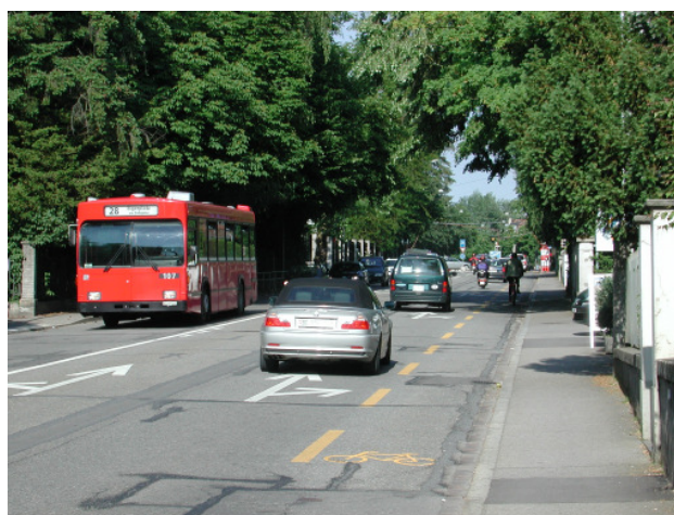
extra-wide traffic lane alongside a cycle lane (Bern)
