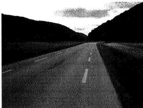
Bargen - Schaffhausen (SH)
