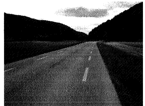
Bargen – Schaffhausen (SH)
