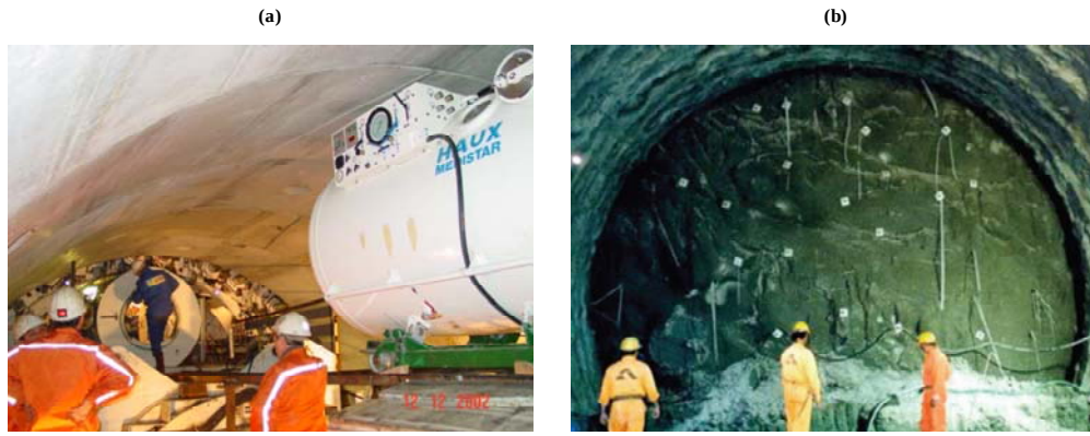
Figure 2.3 Tunnel face support, (a), by compressed air (entrance to the cutterhead for hyperbaric interventions during the construction of the St Petersburg subway, Russia; courtesy of Salini-Impregilo) and, (b), face bolting (bypass Patras, Greece; courtesy of Prof. G. Anagnostou).
