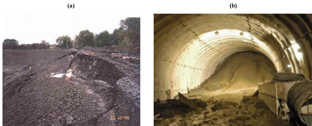
Figure 2.2 (a) Collapse of excavation (after cliffs.lboro.ac.uk/downloads/kovacevic.pdf ) and (b) collapse of a tunnel face (Lausanne subway, Switzerland; courtesy of H. Stadelmann, Implen AG) in weak ground.
