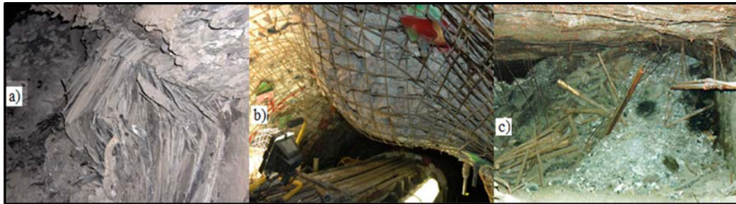
Fig. 1.2 Examples of structurally controlled instability in fault zones: a) highly anisotropic failure at the tunnel sidewalls due to the presence of well-developed foliation or sub-parallel fractures with small spacing; b) progressive block destabilization at the tunnel walls/crown; c) complete collapse resulting from total loss of confinement. After [6].
