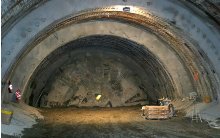
Fig. 1.10 The cutter-head was exposed after more than two years ( http://www.a16.ch ).
