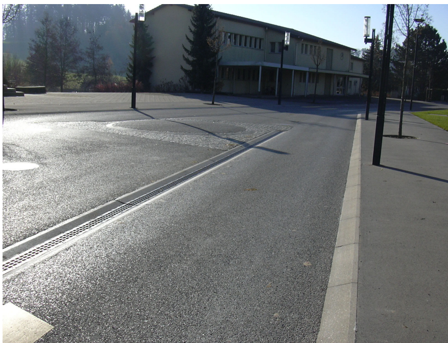
Abb. 6.20: Messung M15 – Route du Centre, Corminboeuf
